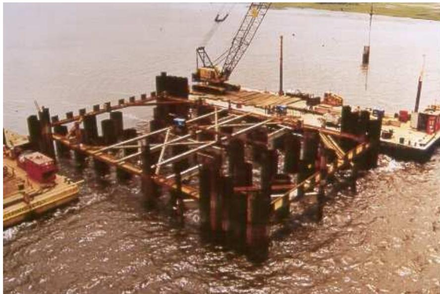
**Figure 11** – Installation of wale and strut system
